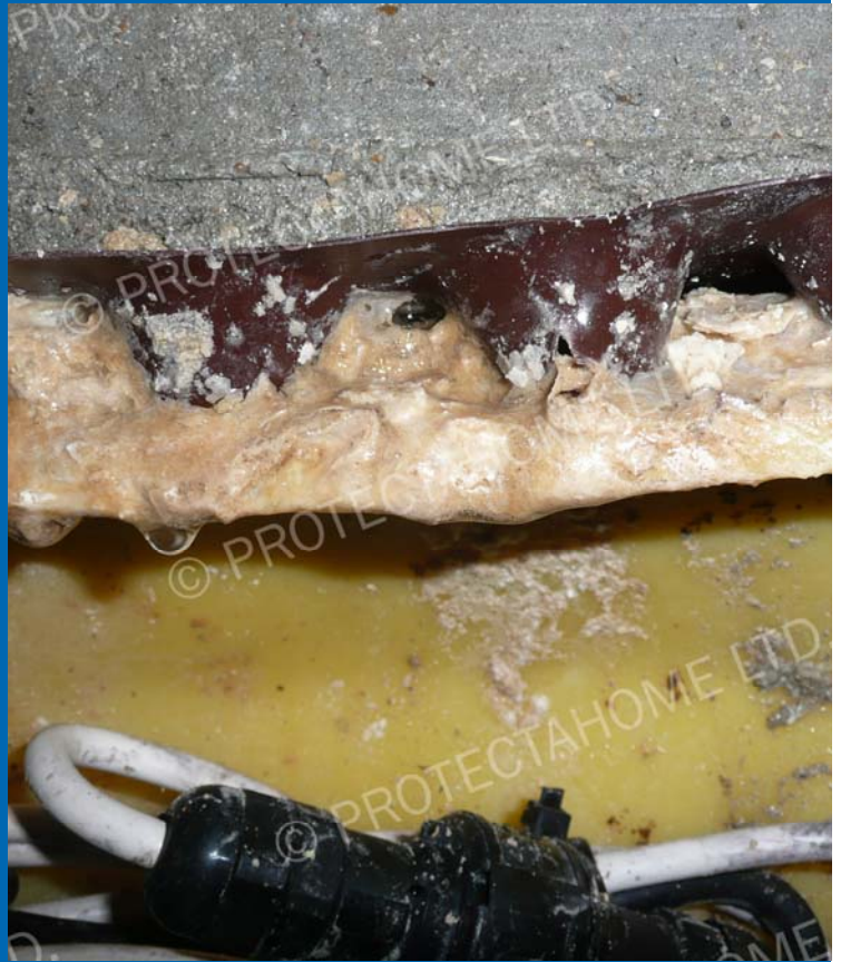
Above: Internal view of a Sump Chamber with connections and membrane entirely blocked by Free Lime.
