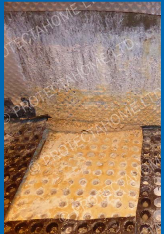
Above: 8mm and 20mm Cavity Drain Membranes after exposure. Entirely blocked by heavy Free Lime deposits.
