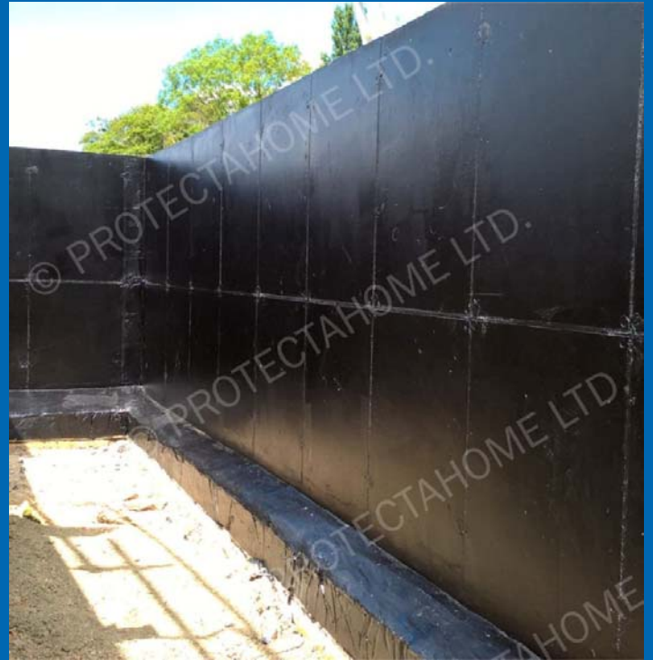
Above: Liquid Membrane applied externally as a Type A (Barrier) Protection System.
