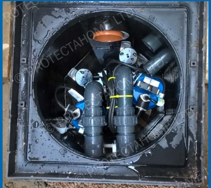
Above: Sump and Twin Pump Installation with Twin Discharge and High Water Level Alarm.
