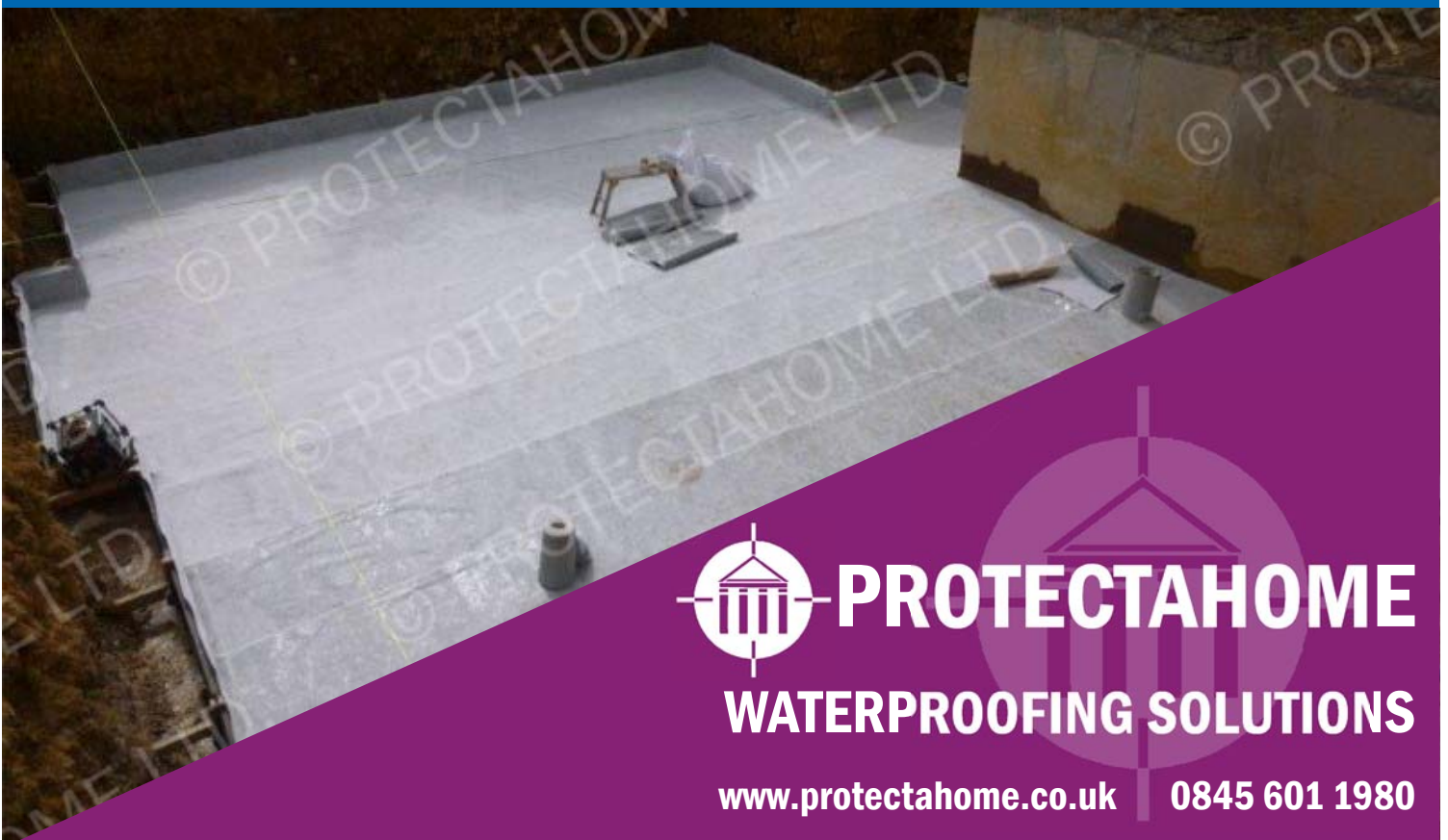
Bottom: Pre-applied Bonded Sheet Membrane installed as Type A (Barrier) Protection System.
